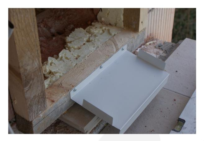
**Frame insulated mounting**, i.e. the doorframe is covered by the thermal insulation of the building:
